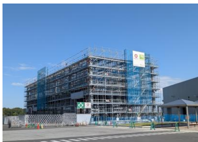
Precious Metals Processing Facility (Under Construction)
